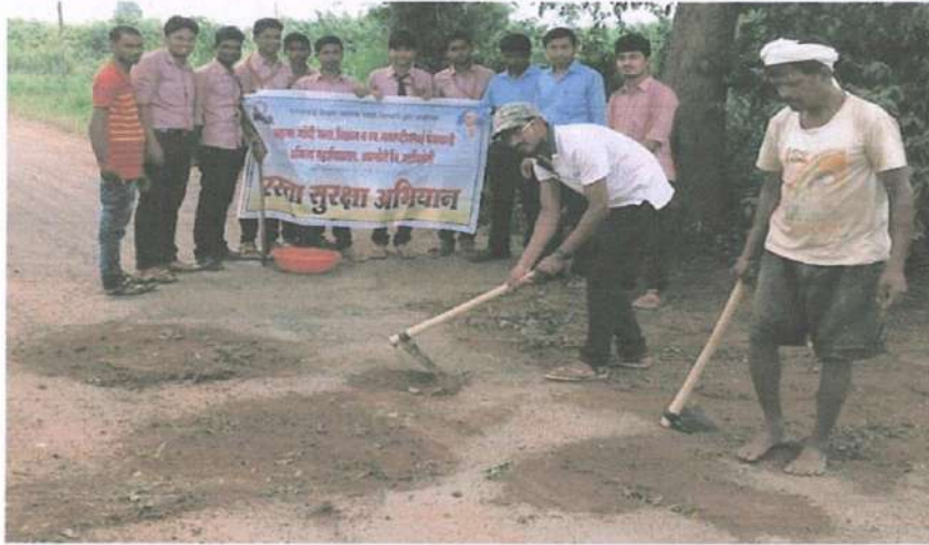
Path-hole filling under Road Safety Drive at adopted village Kasvi – 7 th October, 2016
